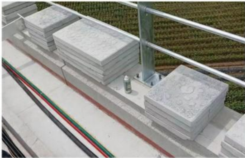
护栏现场安装图 On-Site Installation of Guardrail
