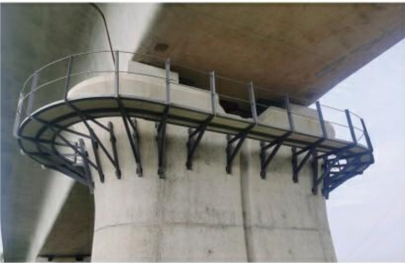
吊围栏现场安装图 On-Site Installation of Hanging Fence
