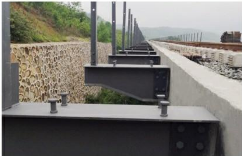
钢横梁现场安装图 On-Site Installation of Goosenecks
