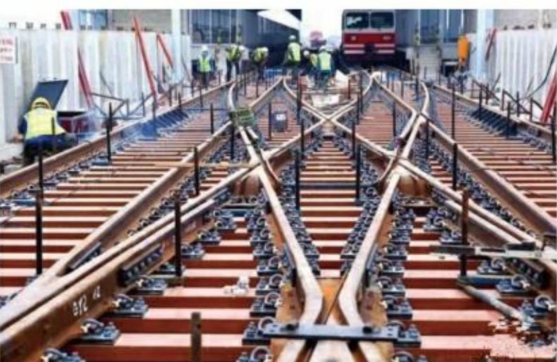
合成轨枕现场安装 On-site Installation of Synthetic Sleepers
