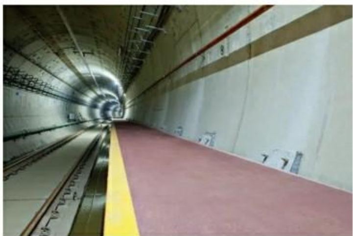
疏散平台现场安装图 On-Site Installation of Evacuation Walkway
